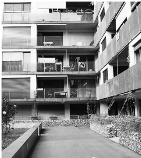
Blick in den Innenhof.
